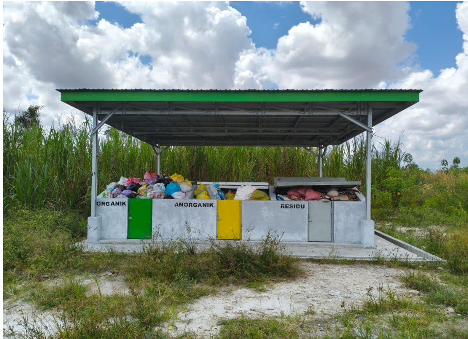
Figure 4. Temporary Waste Collection Point (TPS)
