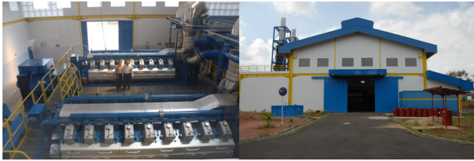
IPP Sarolangun 2 x 7 MW Coal Fires Steam Power Plant (on progress)
