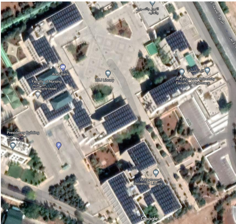
Fig. 2. Satellite google map showing solar panels on top of some buildings in ZUJ
