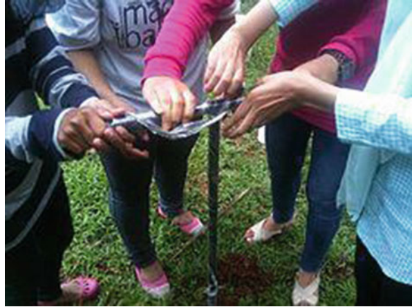
Fig. 4 The making of the biopori H
